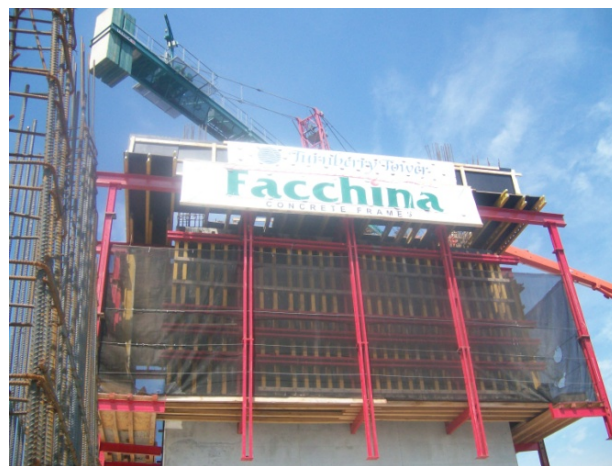
Figure 7.2 – ACS Formwork for Core
