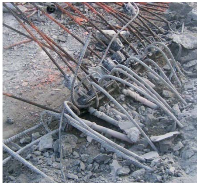
Figure 9.1 - Failed Post Tension Tendons
